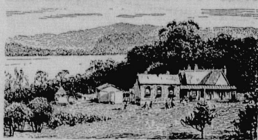
NORTHERN FACADE AND PART OF GROUNDS
