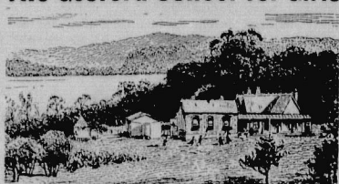
NORTHERN FACADE AND PART OF GROUNDS
